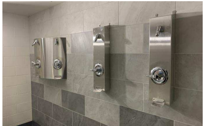
Locker room showers 04/12/2023
