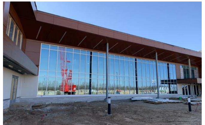
Auditorium lobby glass curtainwall 04/12/2023
