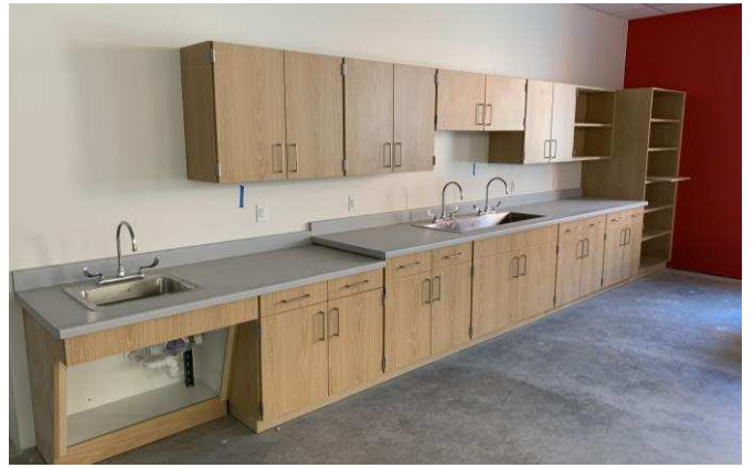
Casework in art rooms 04/12/2023
