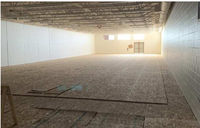
Completed wood subfloor in wrestling room 04/12/2023
