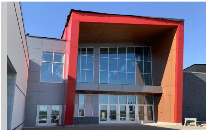
Entrance on South side of building 04/12/2023
